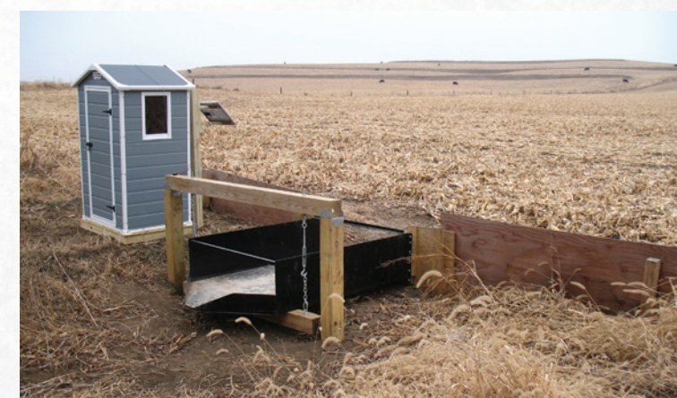
Figure 1. The two-stage flume is placed at the edge of the field to measure surface water runoff. As water moves through the flume, the depth is logged to calculate the volume of water and water samples are pumped into a bucket by equipment inside the shed.
